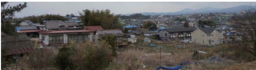
Photo 6.2-54 Damage overview from the east of Minami-machi (Many roofs covered with blue vinyl sheet)
