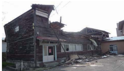
Photo 6.2-18 School building whose 2 nd story collapsed
