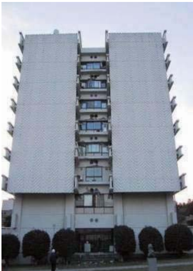
Photo 6.3-27 Appearance of damaged building (Aoba ward, Sendai city)
