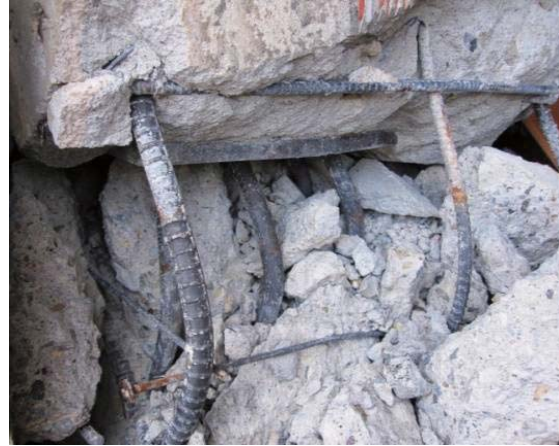
Photo 6.3-26 Close-up view of the bottom of SRC column
