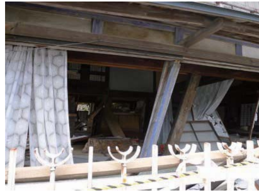
Photo 6.2-32 Inside of the house in Photo 6.2-31
