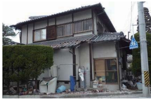
Photo 6.2-49 Damage of roof tile
