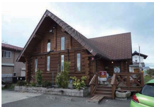
Photo 6.2-27 Log house without damage
