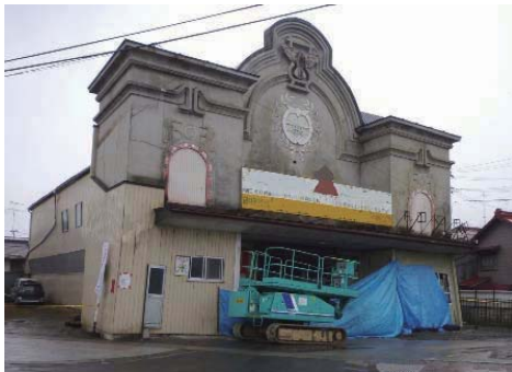
Photo 6.2-5 Large-scale wood building renovated to a factory
