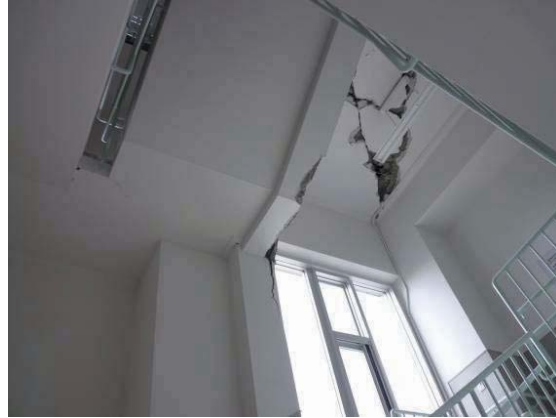
Photo 6.3-36 Bottom of the tower
