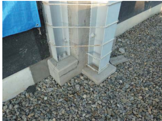
Photo 6.3-11 Column strengthened with H-shaped steel
