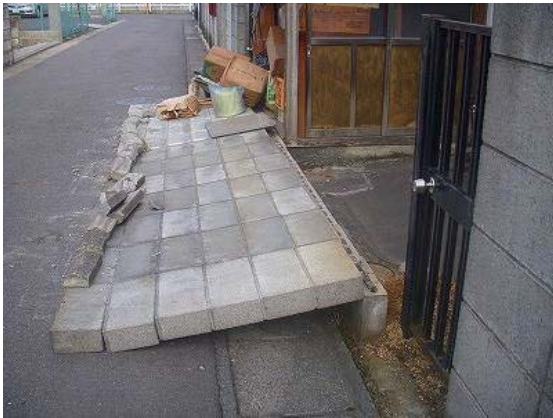
Photo 6.3-50 Collapse of concrete block wall (Koriyama city)
