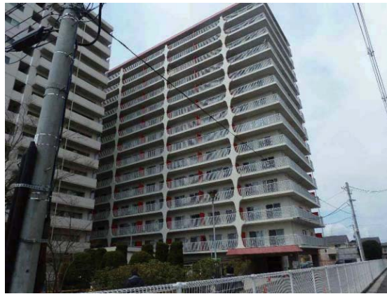
Photo 6.3-29 Appearance of tilted building (Miyagino ward, Sendai city)
