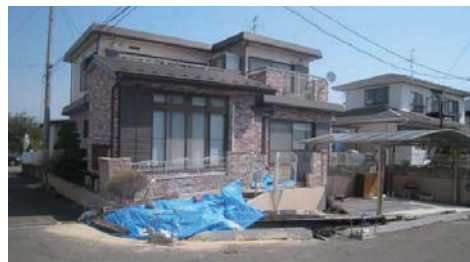
Photo 6.5-16 Houses damaged near the top of hill
