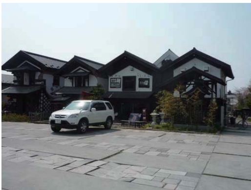
Photo 6.2-11 Warehouse with mud walls damaged heavily or slightly
