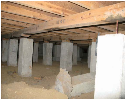
Photo 6.4-13 Overturning of floor strut
