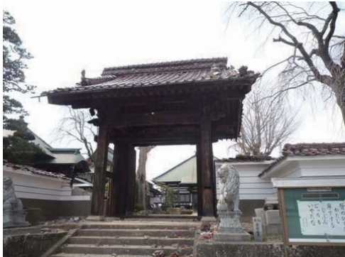
Photo 6.2-50 Minor damage of temple gate
