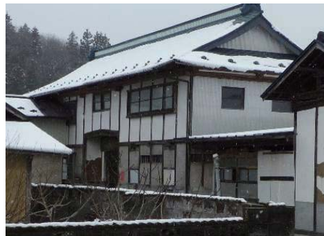
Photo 6.2-8 Drop of mud plasters of Nagaya-mon gate (Kurikomasakurada)
