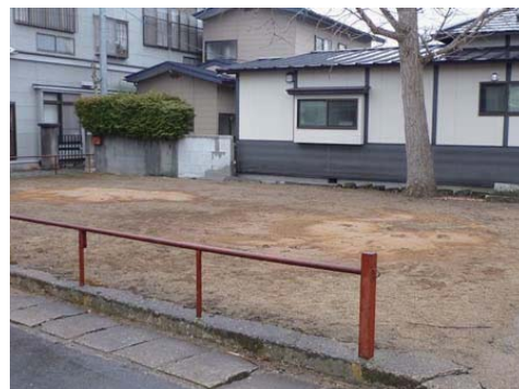
Photo 6.2-2 Sand boil due to liquefaction
