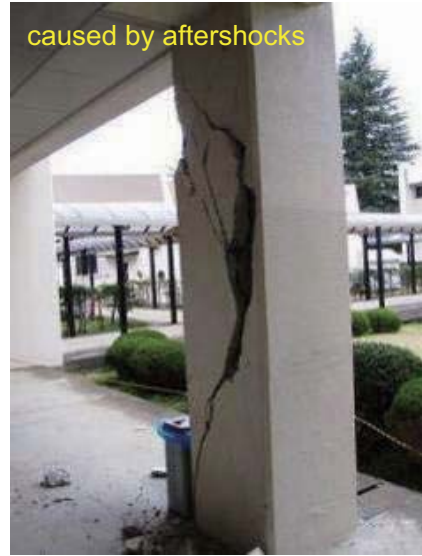
Photo 6.3-13 Shear cracks of first-story columns
