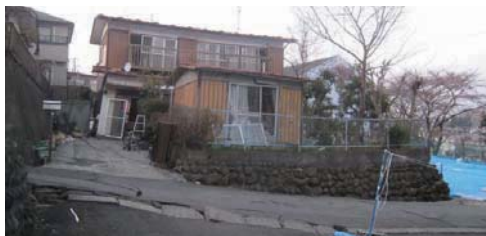
Photo 6.5-15 Damage to houses due to sliding and ground deformation
