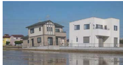
Photo 6.5-7 Damage situations by liquefaction
