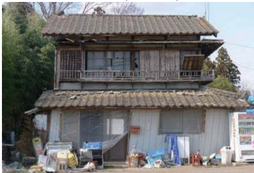
Photo 6.2-74 Damaged house with store (Kadobe)
