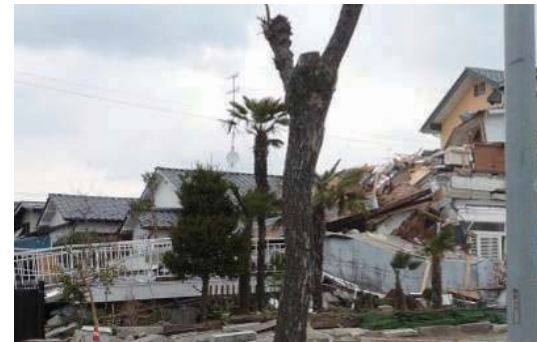
Photo 6.2-53 Collapsed building (Unknown structure type)
