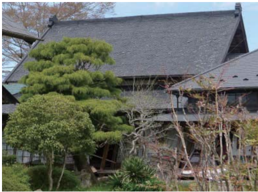
Photo 6.2-31 Heavily damaged house
