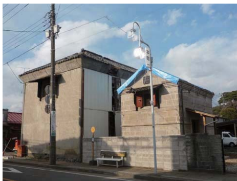
Photo 6.2-55 Damage of stone-built warehouses
