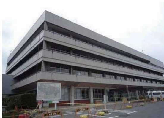
Photo 6.3-14 Appearance of damaged building (Sukagawa city)
