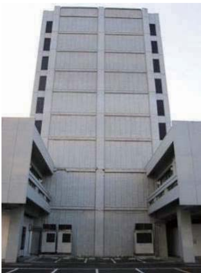
Photo 6.3-20 Appearance of damaged building (Aoba ward, Sendai city)
