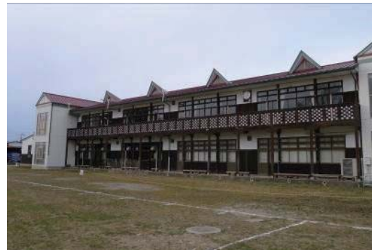
Photo 6.2-79 Wood school building
