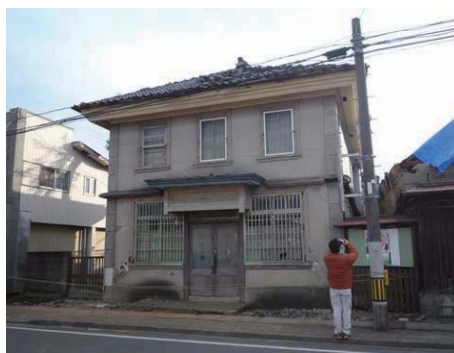
Photo 6.2-56 Damage of an old post office
