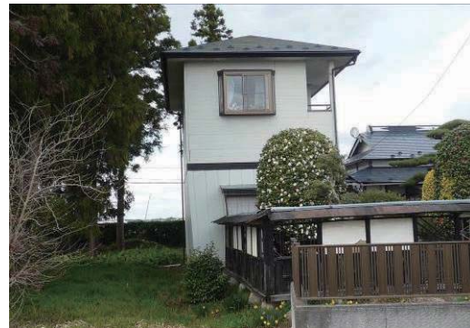
Photo 6.2-26 Tilted two-story house
