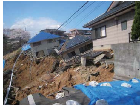
Photo 6.5-18 Land sliding of slope on the southwest of hill and sliding houses
