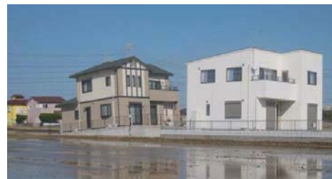
Photo 6.5-7 Damage situations by liquefaction
