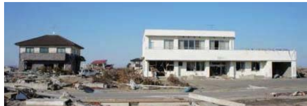
Photo.7.4-7. Wood house remained in the downstream of RC building in Arahama, Wakabayashi ward, Sendai city.
