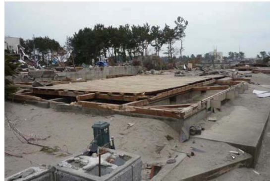
Photo 7.4-15. Fallen Protect forest and wood house (8) washed away in Yuriage, Natori city.
