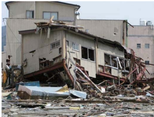
Photo 7.2-10 Story collapse of first floor in a 2-story steel building
