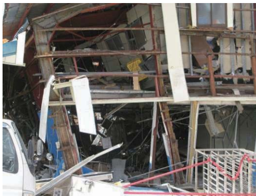
Photo 7.2-11 Tilted gabled roof frame
