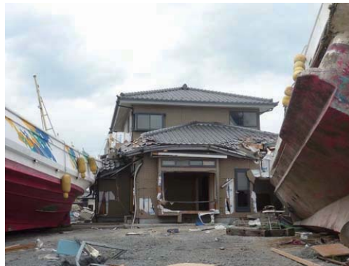
Photo 7.4-26. Wood house remained in spite of ships' crashing in the west of Arahama port.
