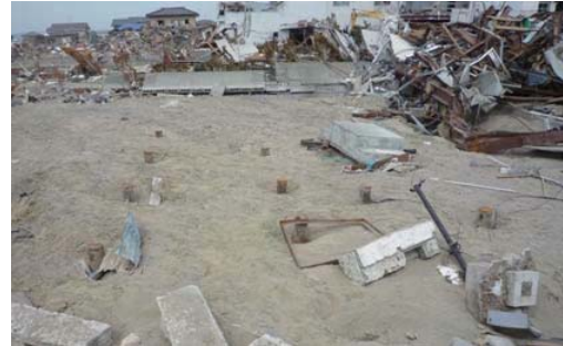
Photo 7.4-11. Steel tube pile left at the the original position ( 2 ) of house in photo 7.4-10.
