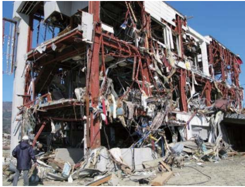
Photo 7.2-12 A remaining 3-story steel building
