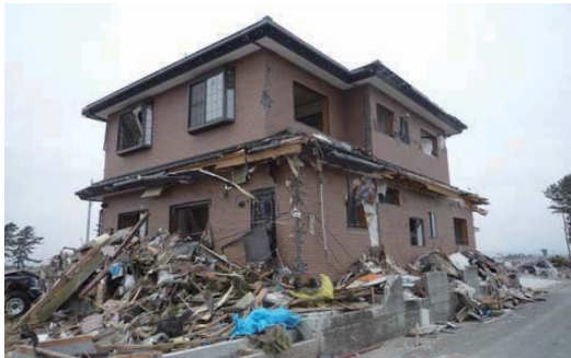
Photo 7.4-18. Japanese conventional post and beam wood house (11) remained alone.
