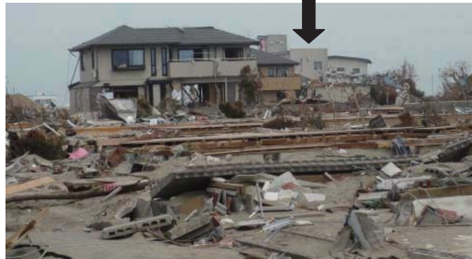
Photo 7.4-21. Wood houses (15) which were not washed away selectively in the downstream of a factory building.
