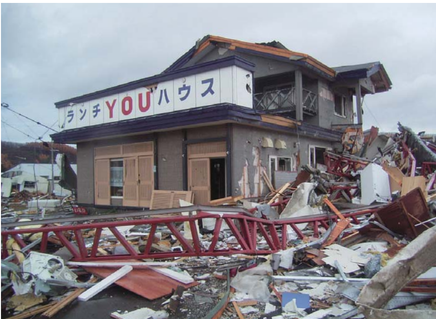
Photo 2. The many objects that turned into flying debris in a major tornado in Hokkaido, November 2006
