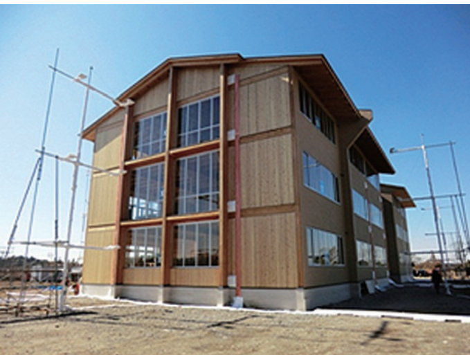
Photo 2: A three-story wooden school building constructed for full-scale fire testing purposes
