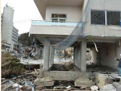
4 storied RC frame building
