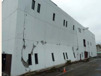
3 storied RC factory building
